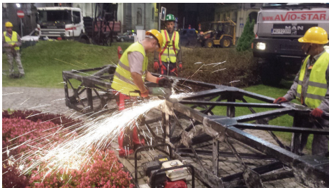
FIGURE 12. ‘Tęczą’ being prepared for transport immediately after disassembly (photo by T. Samseł, August 2015)
