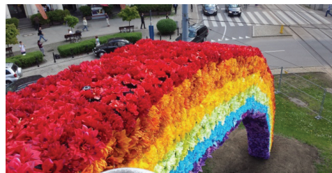
FIGURE 6. Aerial view of 'Tęczą' together with the fire extinguishing system on the day reconstruction was completed after the fire (photo by T. Samsel, April 2014)
